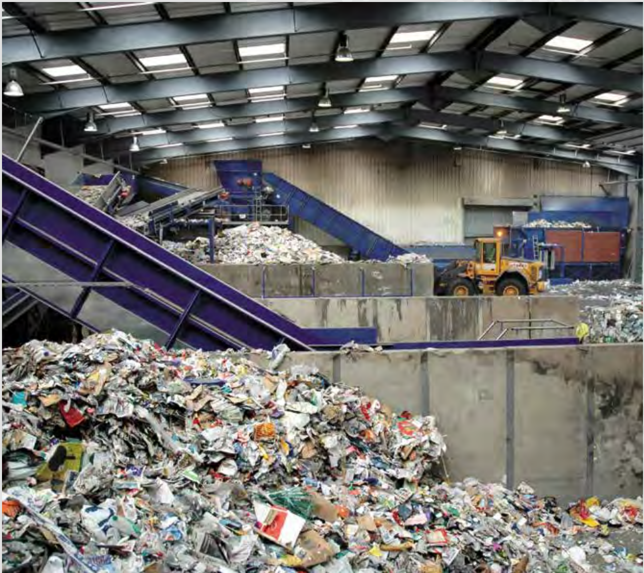
Reppie waste-to-energy plant, Addis Ababa, Ethiopia Photo credit: © The Kenyan Wall Street
