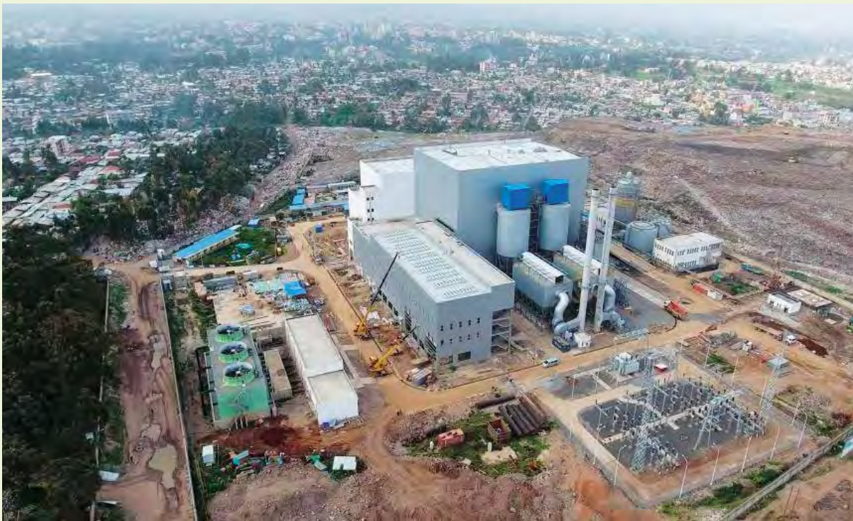
Reppie 50MW waste-to-energy plant at the Koshe dump in Addis Ababa, Ethiopia
