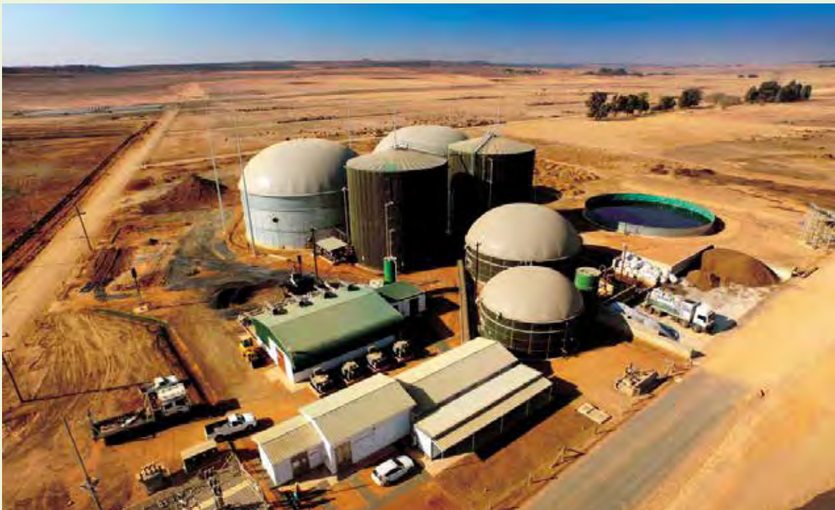
Bio2Watt biogas plant, Bronkhorstpruit
